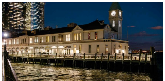
Pier A Harbor House | Private Event Space Battery Park
